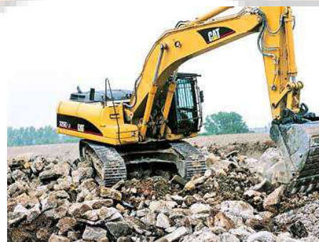
Fig. New Power Shovel
